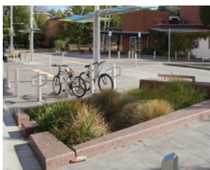
Examples of WSUD (From top to bottom) at the UC Innovation Centre and Childers Street, Acton (Photos courtesy of Luke McPhail)
